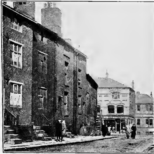
SLIDE No. 28.—CONDEMNED PROPERTY IN HOWELL CROFT NORTH.
